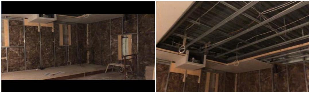
The fibre optic ceiling was created by me. Using black plywood, we were able to create the star ceiling effect relatively easily. This was achieved simply by drilling tiny holes in to the plywood and threading the fibre optics through the drill holes. We then used a blue led trim around the edge to give a deeper light effect. These were then connected to the control 4 system.
